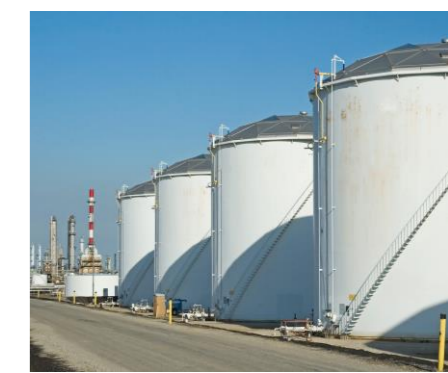
Oil Storage Tank
